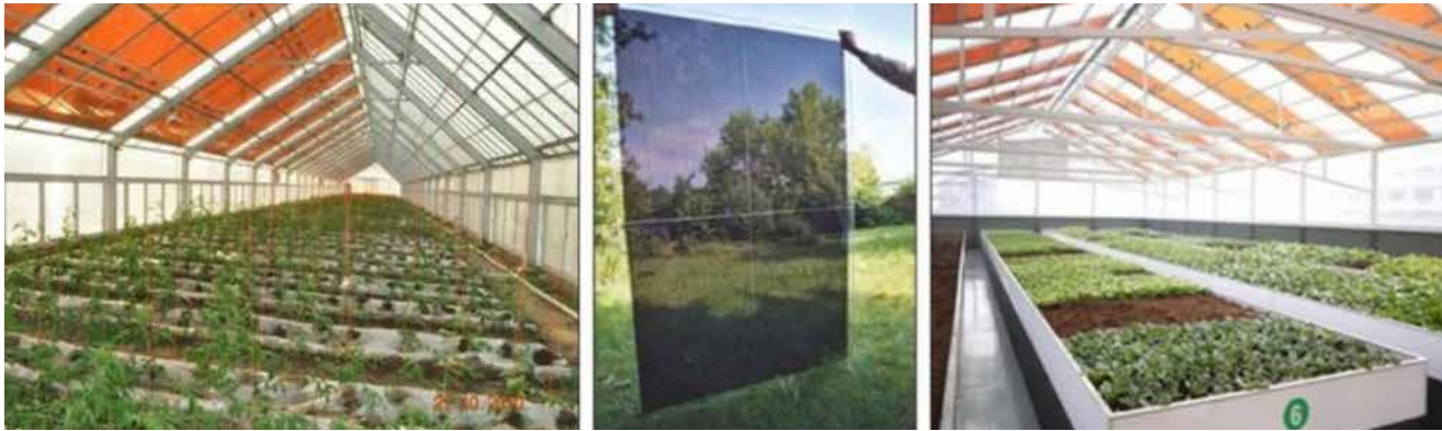
1. Semi-transparent solar module roof type structure
